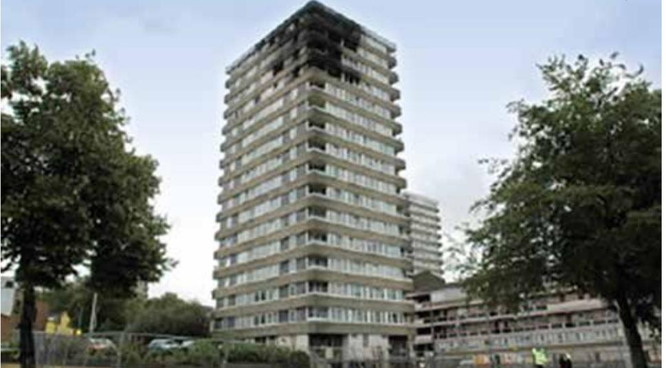
Conducted for the Department of Communities and Local Government (DCLG), 'Fire safety issues with balconies' found that methods deployed to meet Part L of the building regulations – such as improving insulation and preventing thermal bridging – may be compromising fire safety as stipulated by Part B.
